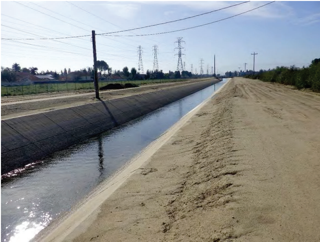
Photograph 3. South-facing view of the Arvin-Edison Canal within the eastern portion of the survey area (35.349586°, -119.096725°).
